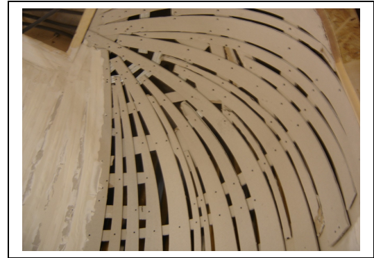
Figure 6: Construction of the domed ceiling
