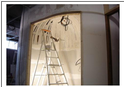
Figure 5: Construction. Outside view
